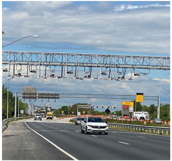
All Electronic Tolling (AET) at the Bay Bridge
