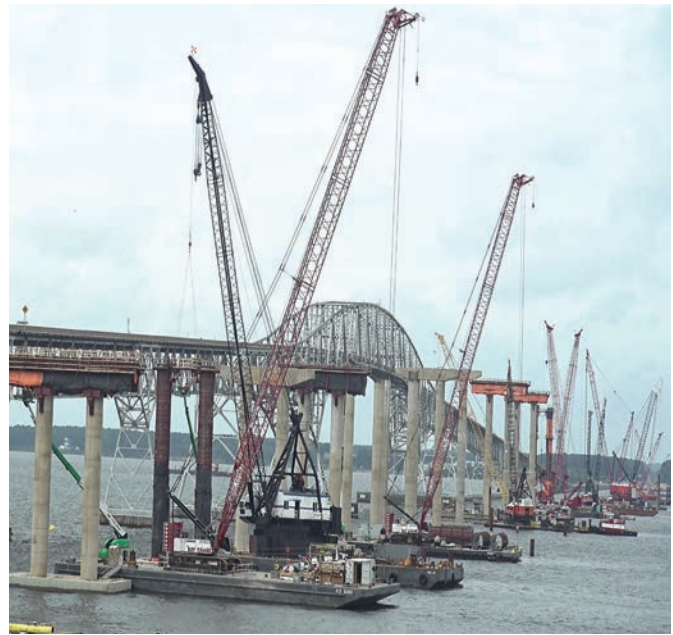
New Nice/Middleton Bridge Project
