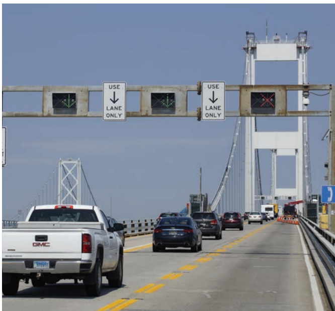
Westbound Bay Bridge Rehabilitation
