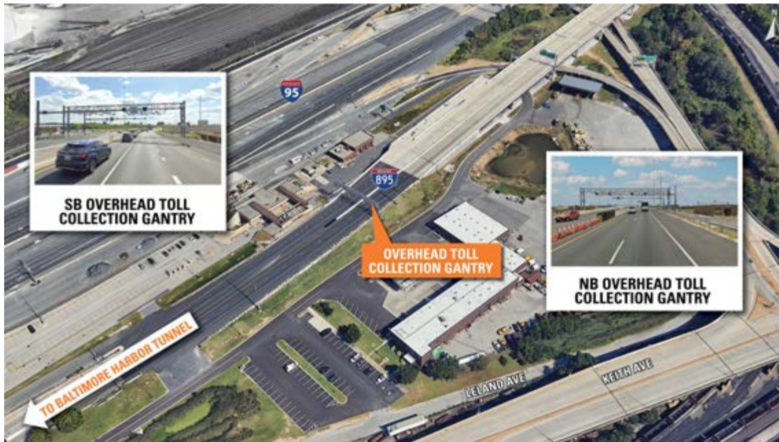
Overhead Toll Collection Gantry - North of Harbor Tunnel
